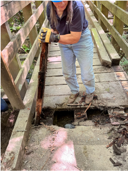
Blanchard DNR National Trails Day work party, June 3, 2023 pictures. Fixing bridge.
